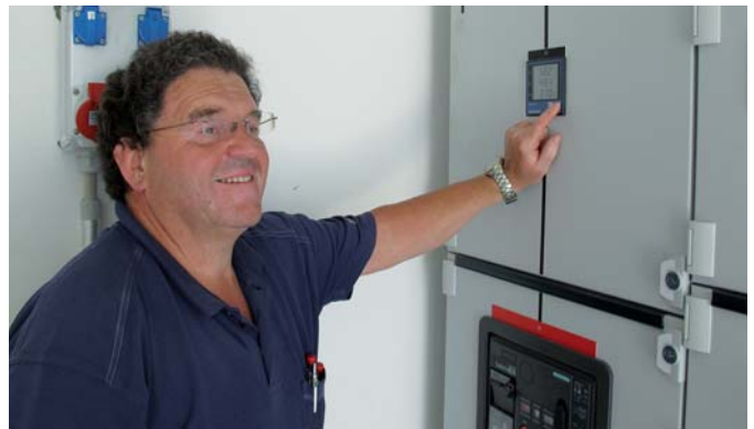
Laboratory IT system supply and MK2430 indicator unit
